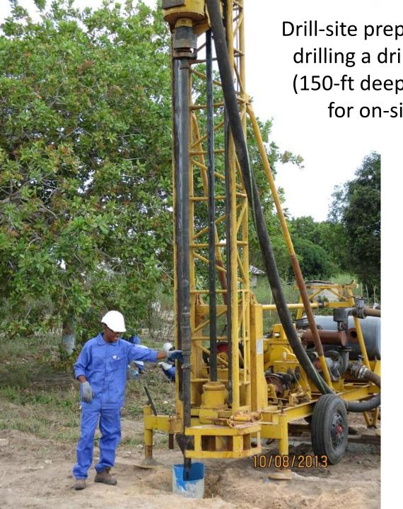
Drill-site preparations included drilling a drinking water well (150-ft deep, 2-in diameter) for on-site water use
